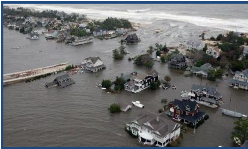
Hurricane Sandy coastal flooding in Mantoloking, NJ. Photo Credit: New Jersey National Guard/Scott Anema.
