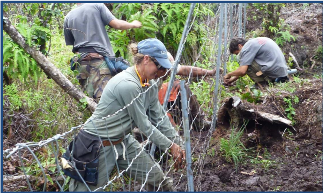
Hawaii's Watershed Partnerships construct fences in critical natural areas to protect natural resources and ecosystem services from the impacts of invasive animals. Photo Credit: Emma Yuen, Hawaii Department of Land and Natural Resources.
